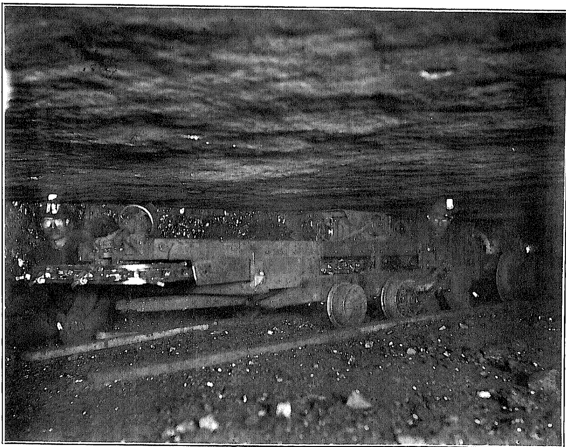
PLATE III.—ELECTRIC COAL CUTTER.
