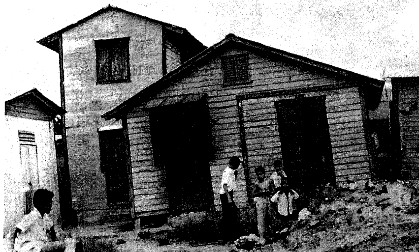
Figure 16. Sometimes whole houses sag. Both of these are dilapidated.
