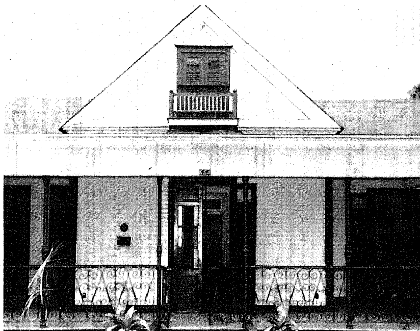
Figure 1. A sound house may have no visible defects or only slight defects that are easily taken care of by regular upkeep.
