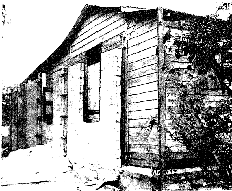
Figure 21. When units are being rebuilt or repaired, judge the condition of the original structure, not the part under construction. For example, a deteriorating house continues to be deteriorating until the reconstruction or repairs are completed.
