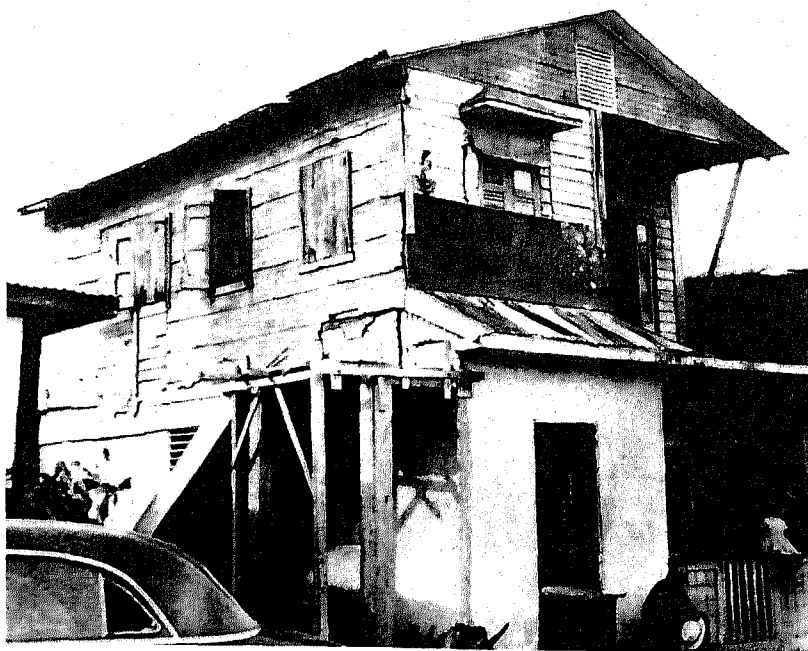
Figure 22. When multiunit structures are being rebuilt, judge the condition of the entire structure, and mark all units accordingly. The makeshift material used in this house shows it is of inadequate original construction.
