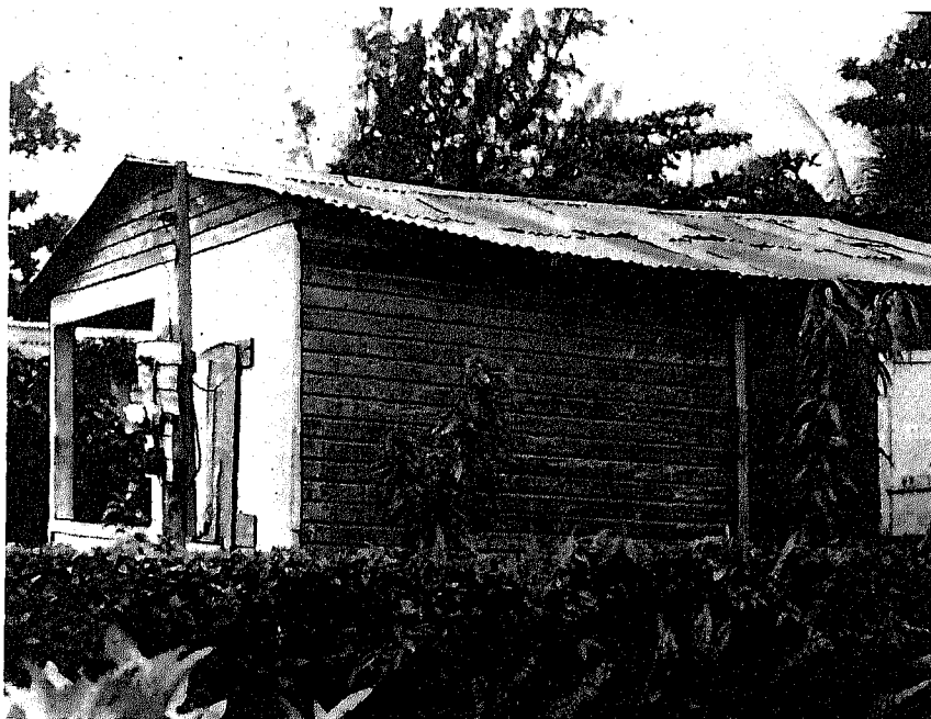
Figure 15. Noticeable sagging is a critical defect. A sagging roof is evidence that the supporting walls have settled.
